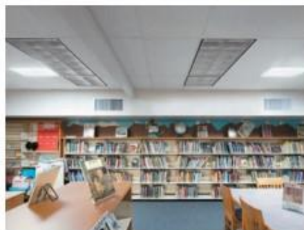
The Douglas County School District added daylight to several of their K12 facilities with help from Solatube.
